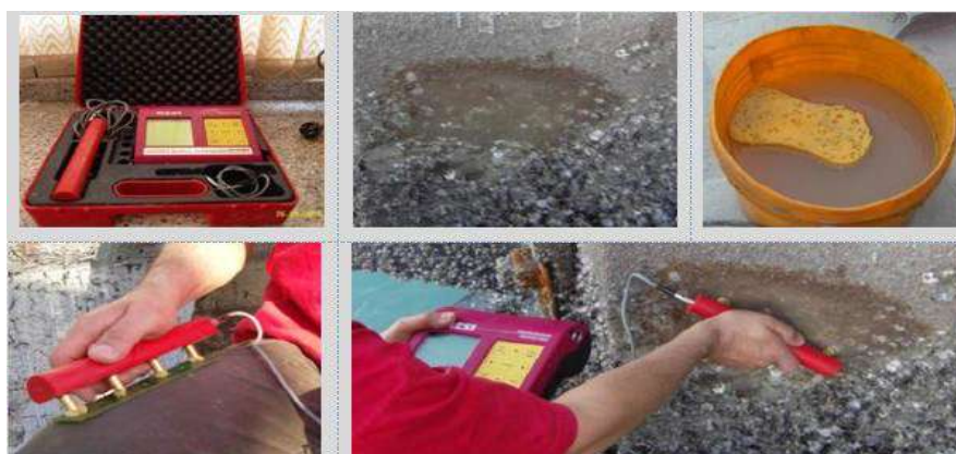
Fig. 6. A view of the concrete superficial electrical resistivity test performed by using the Wenner method on the concrete pier
