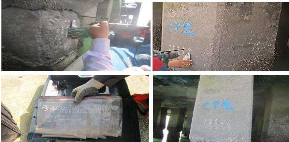
Fig. 3. Concrete drilling to get concrete powder
