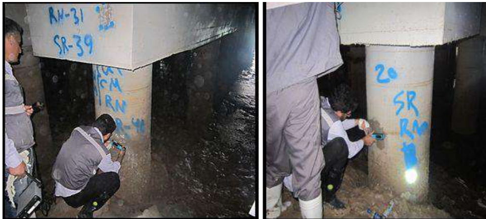
Fig. 7. Concrete electrical resistivity test on Piles docks 11 and 12
