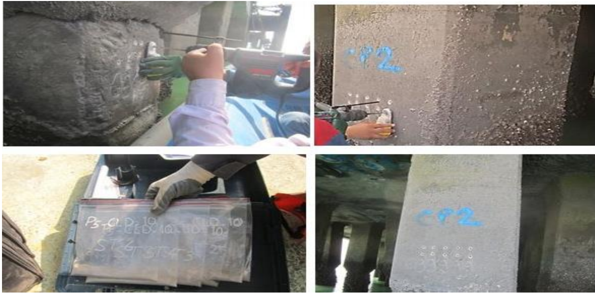
Fig. 3. Concrete drilling to get concrete powder
