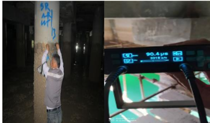
Fig. 8. Concrete ultrasonic test on piles, slabs and forehead at Piers 11 th and 12 th
