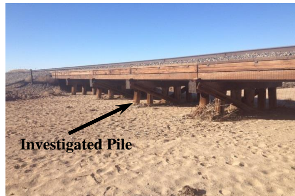
Fig. 15. Street view of bridge with superstructure and investigated pile
