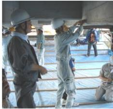
①Preparing damage sheet drawings
