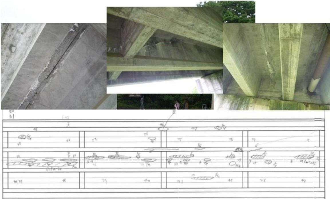
Fig. 6. Damage situation of the target bridge and the damages identified by an inspector
