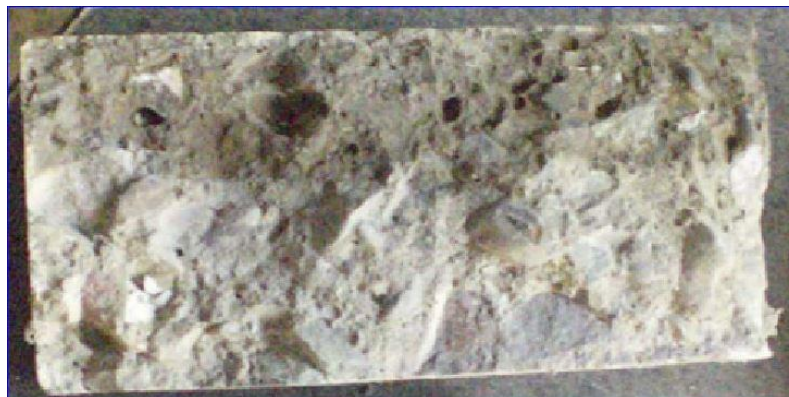
Fig. 3. Color change of concrete sample section after silver nitrate spraying
