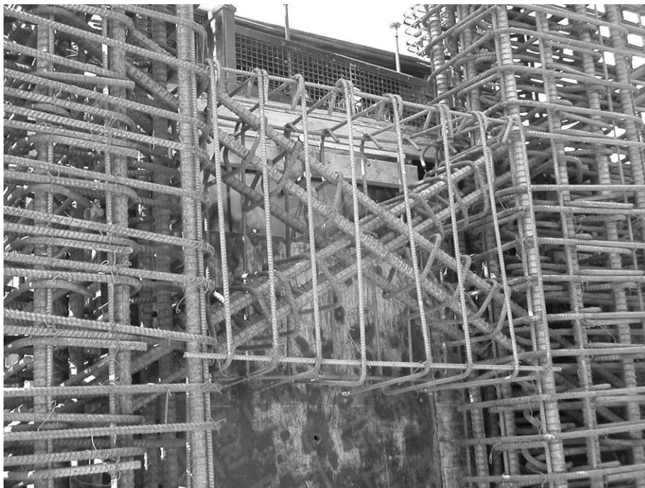
Fig. 9. Diagonal reinforcement bracing in spandrel beam
