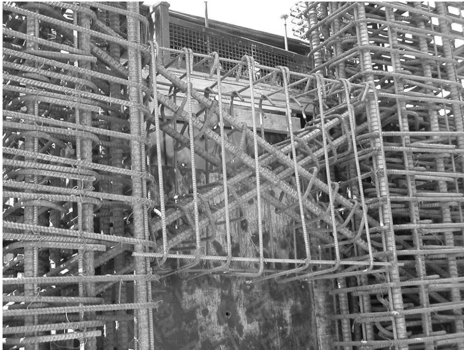
Fig. 9. Diagonal reinforcement bracing in spandrel beam
