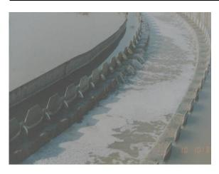
**Fig. 3.** Sample of unsuitable construction work (unbalanced V-notch) (Amirtaimour, 2008).
