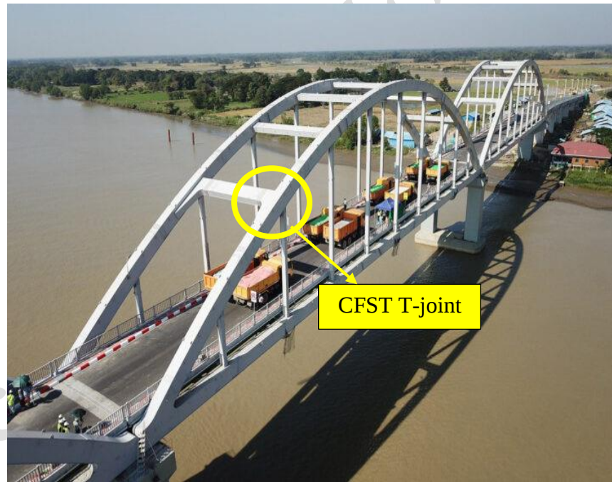
Figure 1. Overview of the CFST T-joint used in the bridge structure
