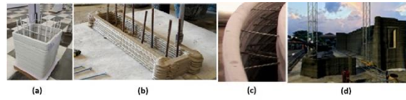
Fig.14. Reinforcement methods for printed concrete include techniques adopted by: (a) (WinSun, 2021) WinSun, (b) (CyBe, 2022) CyBe, and (ApisCor, 2018) Apis Cor. (d) Construction of a concrete building in real dimensions and armed with this method.
